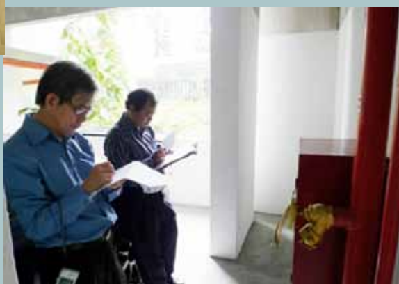
Knight Rider Auditor and Condominium Manager noting down a fire hydrant's defects.
