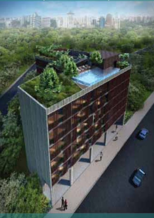
Killiney 118 - View of the Rooftop
